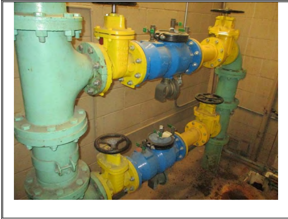
BACK FLOW PREVENTION DEVICE (TYPICAL)
