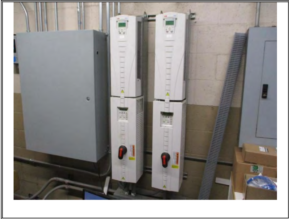
VARIABLE FREQUENCY DRIVES (TYPICAL)
