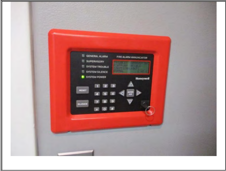
FIRE ANNUNCIATOR SYSTEM (TYPICAL)
