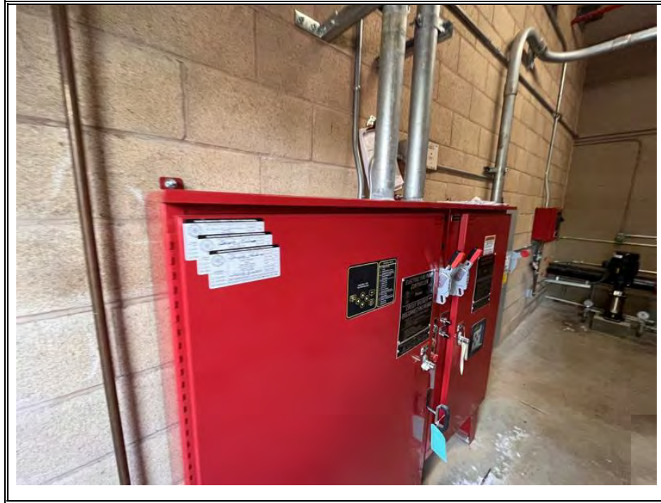
FIRE PUMP CONTROLLER (TYPICAL)
