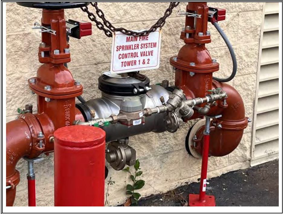
BACKFLOW PREVENTION DEVICE-FIRE LINE (TYPICAL)
