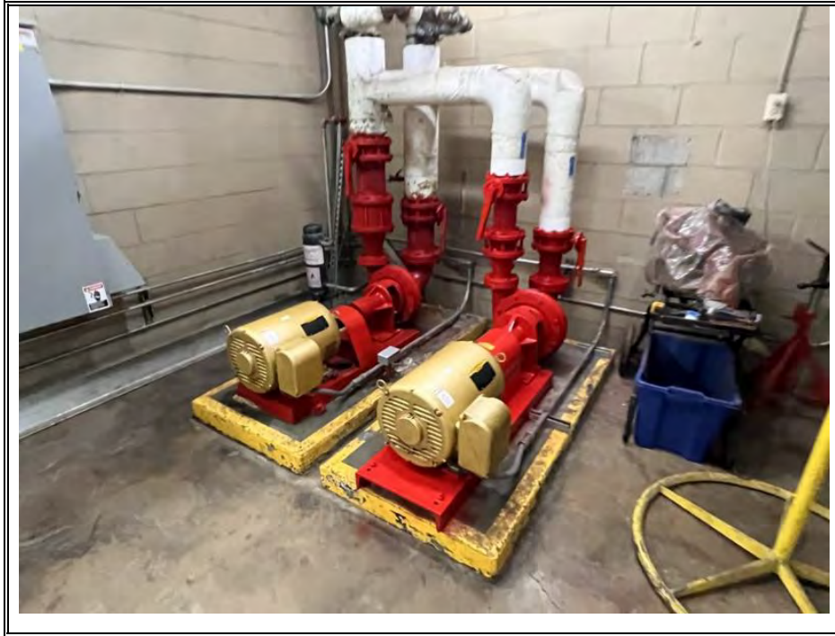
CENTRIFUGAL PUMPS (TYPICAL)
