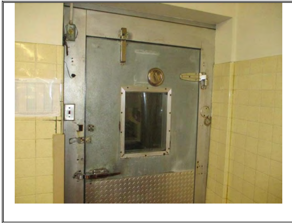
PREFAB WALK-IN FREEZER (TYPICAL)
