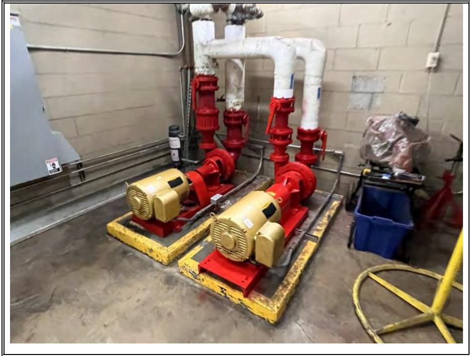
CLOSED LOOP PUMPS (TYPICAL)
