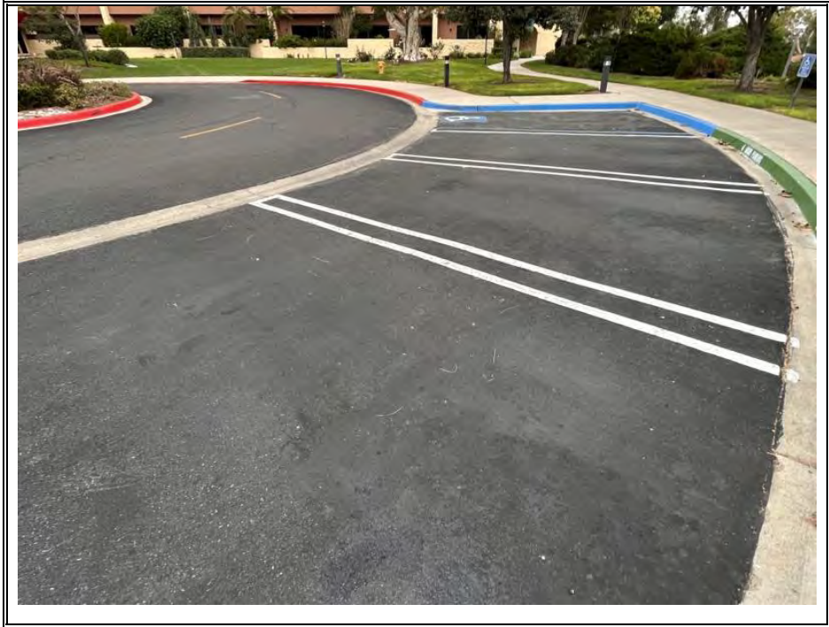
ASPHALT SEAL COAT-NEWER (TYPICAL)
