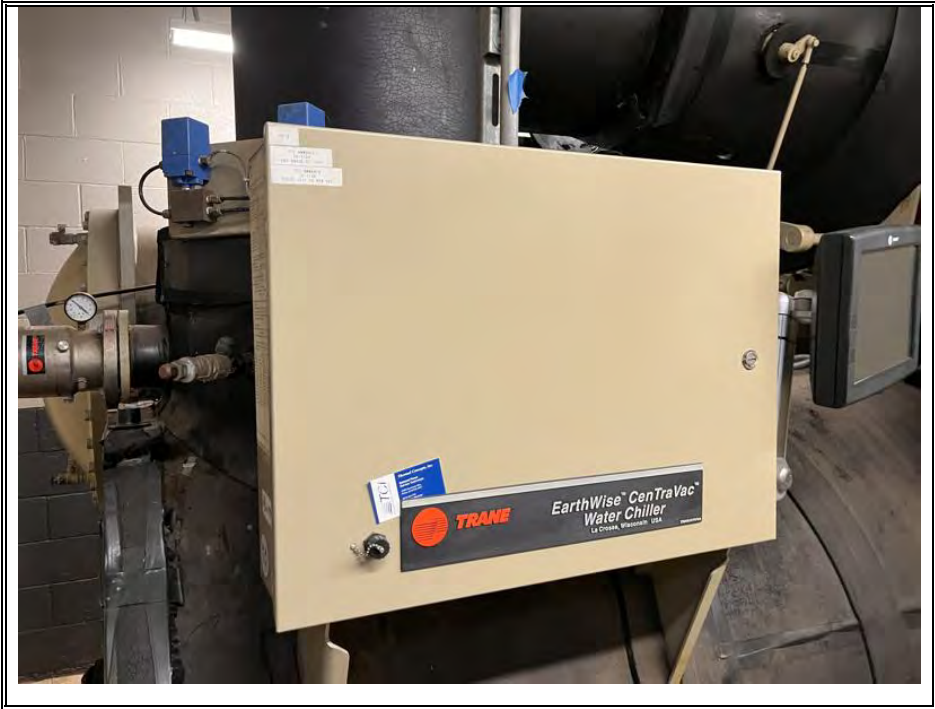
ADAPTIVE FREQUENCY DRIVE (TYPICAL)
