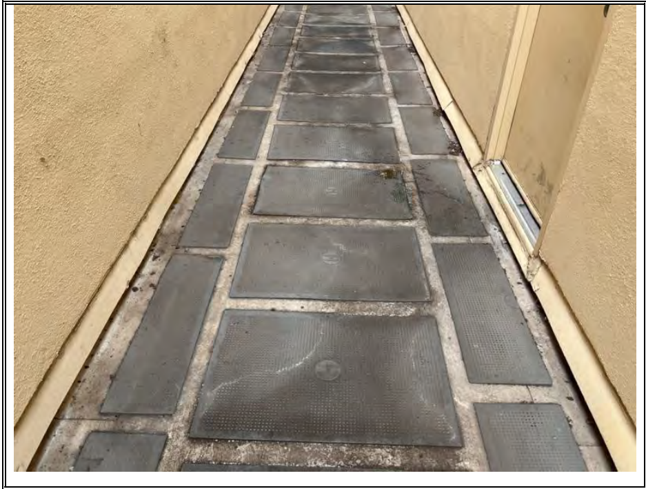
MODIFIED CAP SHEET ROOF (TYPICAL)
