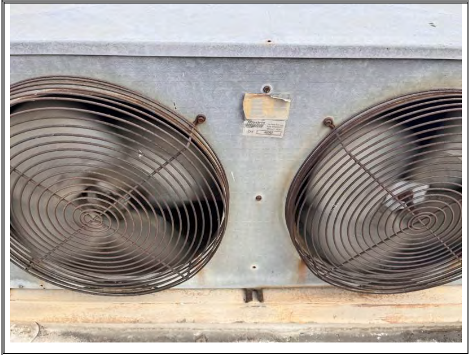
REMOTE AIR COOLED REFRIG CONDENSER (TYPICAL)
