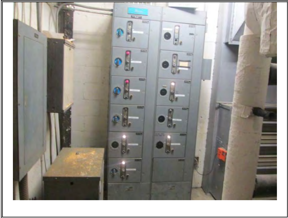
MOTOR CONTROL PANEL (TYPICAL)
