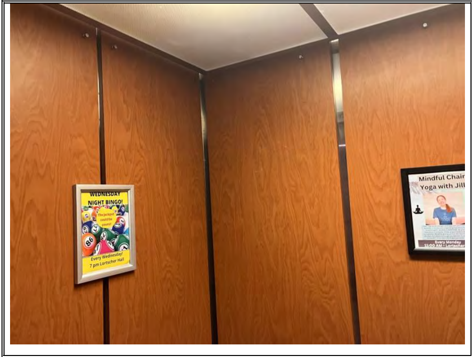
ELEVATORS-CAB REMODEL (PHASE 1) (TYPICAL)
