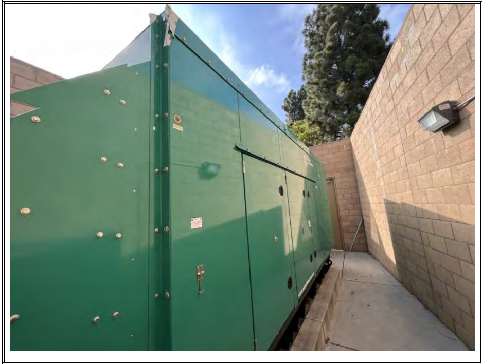
FUEL STORAGE TANK-GENERATOR (TYPICAL)
