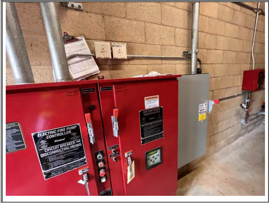
AUTOMATIC TRANSFER SWITCH (TYPICAL)
