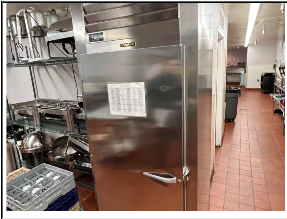
SELF-CONTAINED REACH-IN REFRIG UNIT (2019) (TYPICAL)
