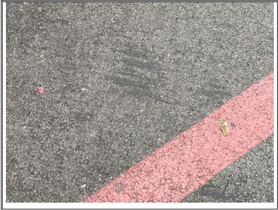
ASPHALT SEAL COAT - OLDER (TYPICAL)
