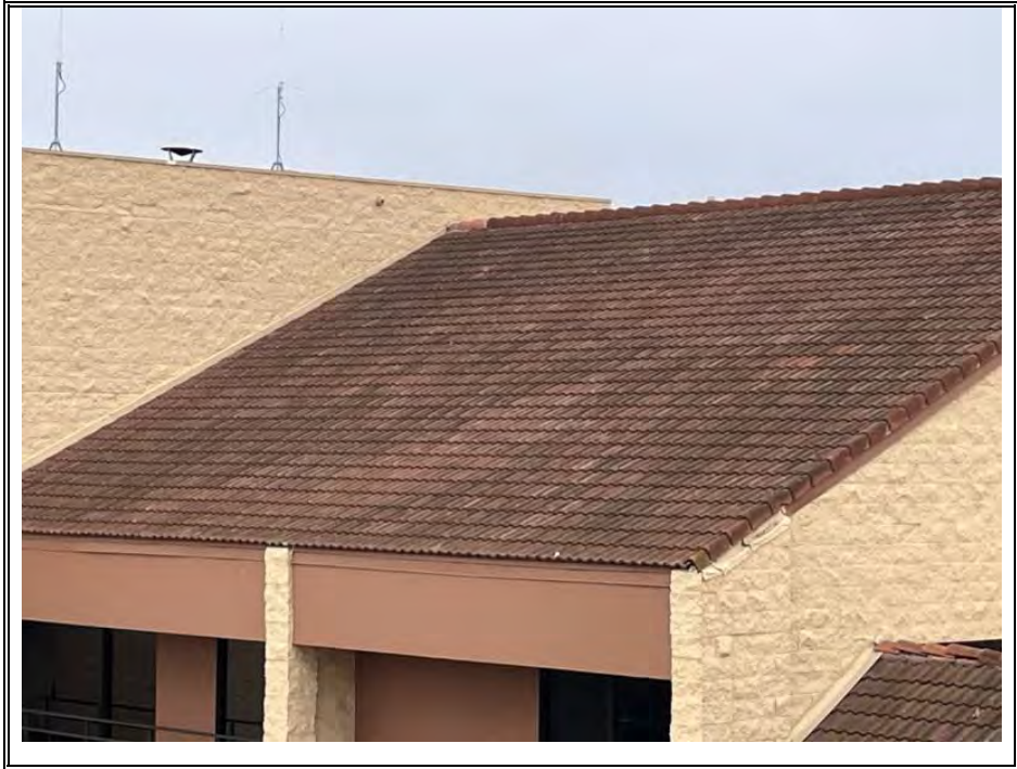
CONCRETE TILE ROOF (TYPICAL)
