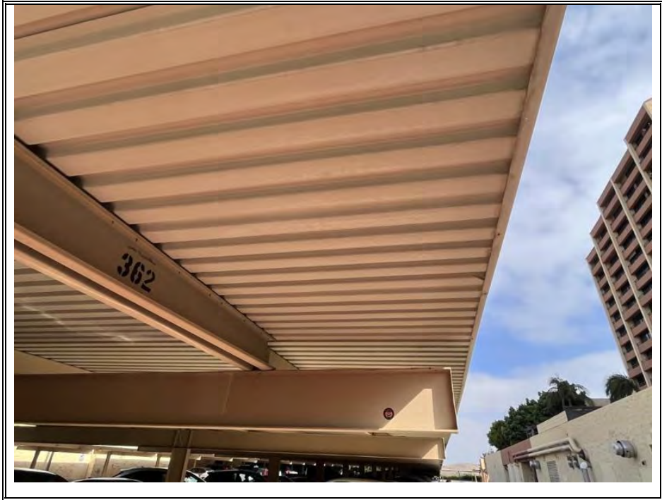
IRONWORK-EXTERIOR (GROUNDS) (TYPICAL)
