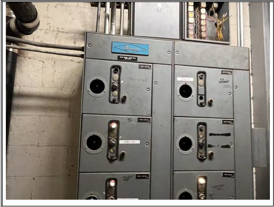
MOTOR CONTROL PANEL (TYPICAL)
